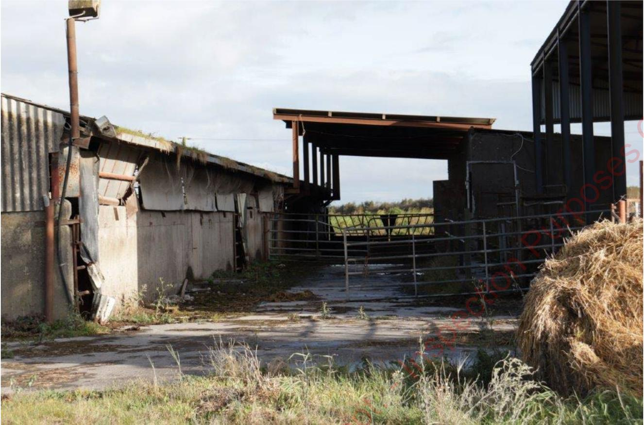
**Plate 4-7:** Adjacent four bay agricultural shed unit with steel cladding roof
