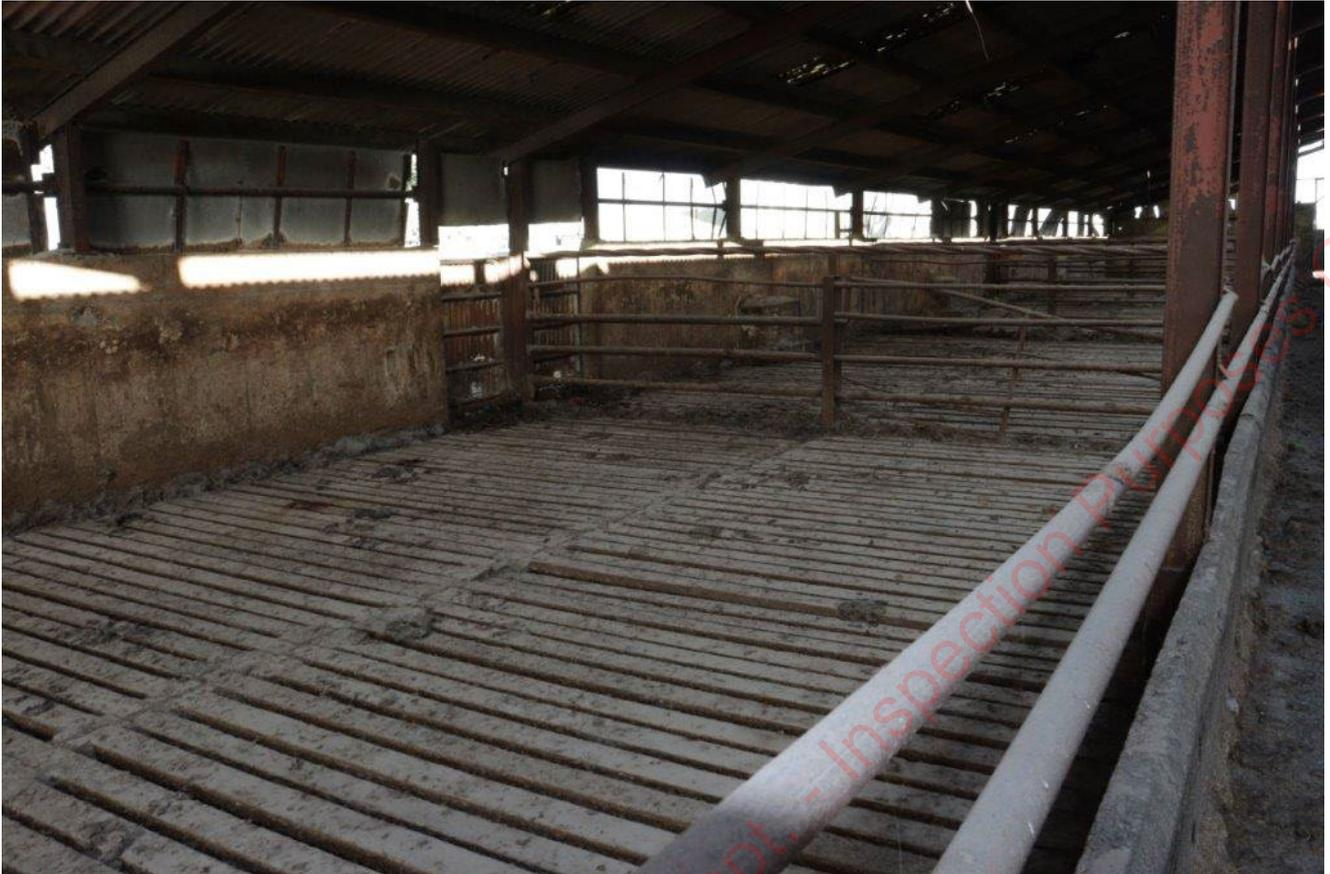
**Plate 4-5: Concrete Slatted Floor of Main Agricultural Shed Unit**
